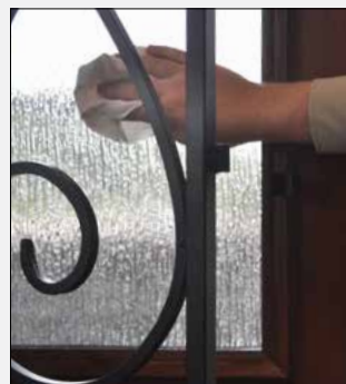
Operable wrought iron grilles
