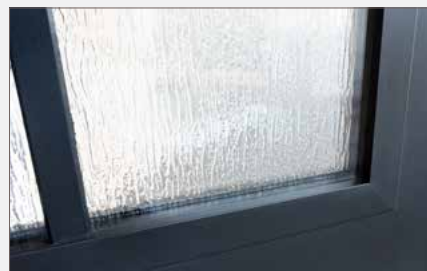
Aluminum glass frame provides a flat minimalist appearance on both sides of the door.
